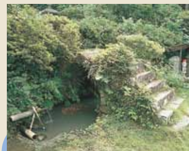
福厳寺羅漢橋 Fukugonji-rakan Bridge
